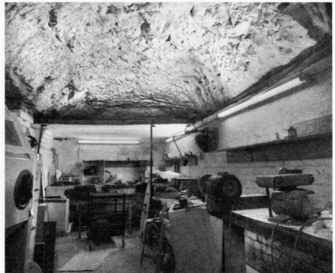
Although most of the tunnels are lined, either in brick or corrugated metal, some areas remain unlined like this workshop in the centre of the complex.
